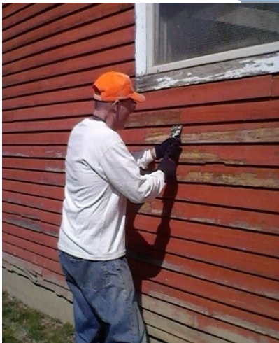
Getting the barn ready for a new coat of paint.
