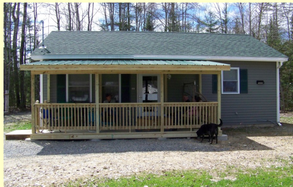
Brent's newly renovated home
